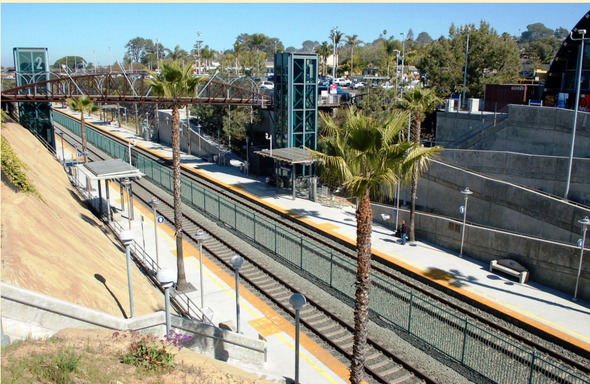
Trench in Solana Beach - Do we want this?
