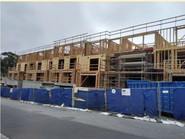
Picture of the new hotel a few weeks ago. The construction of the concrete underground parking took over a year.
